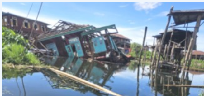
Damaged Home at Inle Lake
