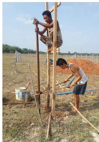
Drilling water well
